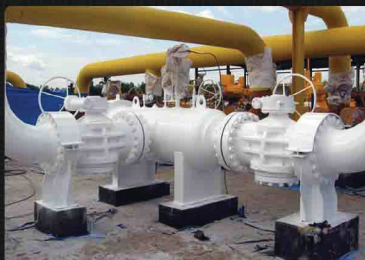
Gas Pipeline - Indonesia
