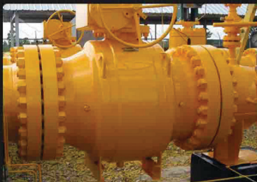
Gas Pipeline - Indonesia
