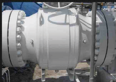
Gas Pipeline - Indonesia
