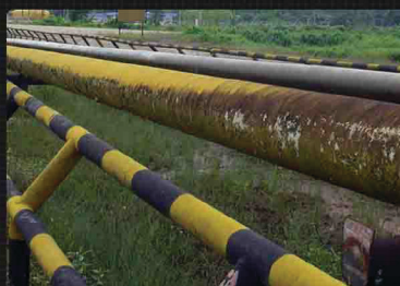
Gas Pipeline - Indonesia
