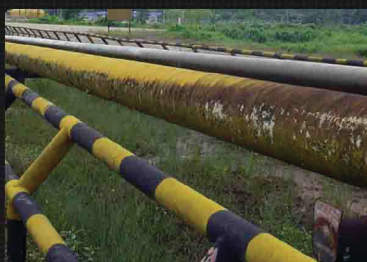
Gas Pipeline - Indonesia
