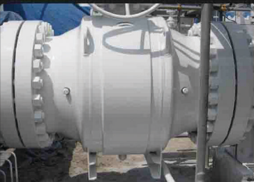
Gas Rohr - Indonesia
