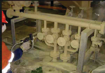
Steam Pipes - Turkey [after]
