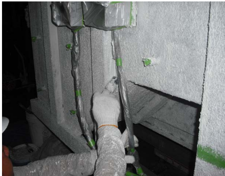
HSC application Third coat
