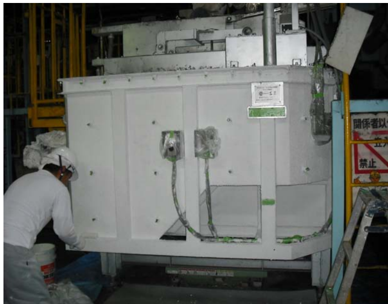
HSC application Forth coat
