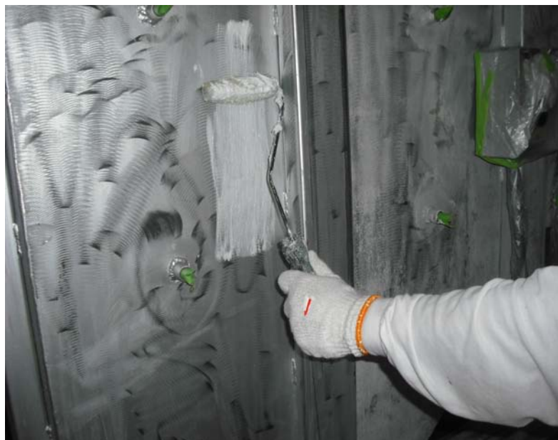
HSC application First coat
