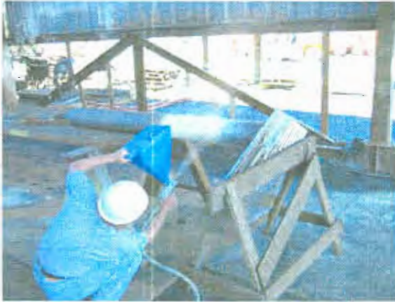
A temperature reduction from 370C on the bare pipe to 90C after the second primer coat @ 50 mils DFT was applied. ( Video )
