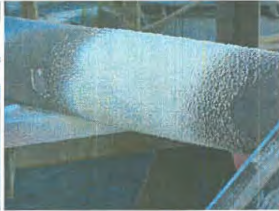
A temperature reduction from 370C on the bare pipe to 90C after the second primer coat @ 50 mils DFT was applied. ( Video )
