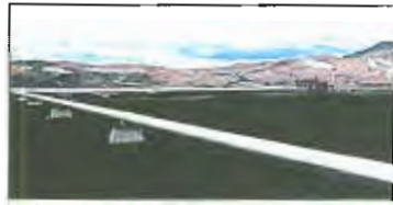
Steampipe from well to Power station
