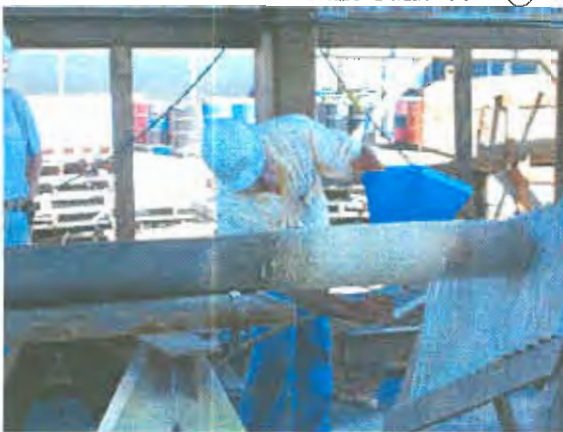
A temperature reduction from 400C on the bare pipe to 50C after the final build coat @ 250 mils DFT TOTAL was applied.
