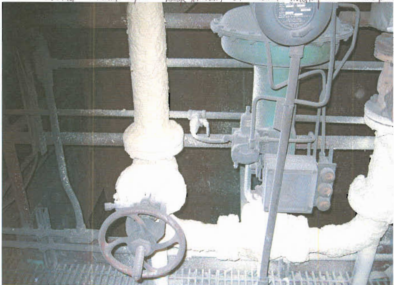
Coated Steam Pipe - Large amount of steam - holding heat - more pressure
