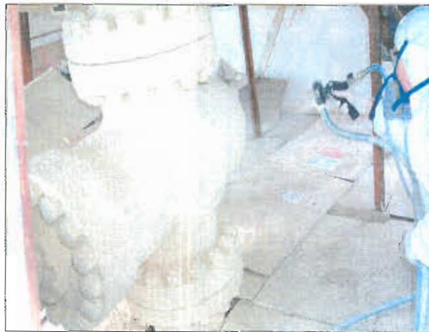
HPC sprayed onto hot surface of the well head
