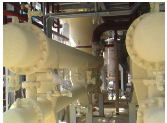
<Condenser (Heat Exchanger)>
