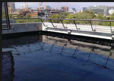
Roofing - Chile [after]
