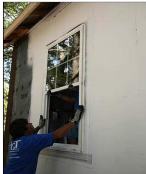
The exterior is clad with James Hardie fiber-cement siding. Windows and doors are installed into pre-cut openings with a minimal use of wood framing. Doors are hung and the roof is shingled, leaving the house ready for furnishing. "Within 60 days we had our house ready for all the interior stuff," says Locklair. "Within 30 more days it was completely finished."
